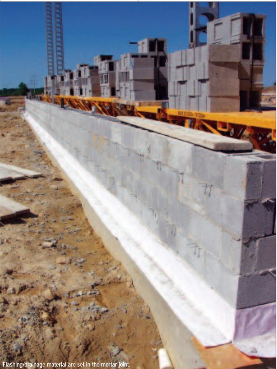
Flashing/drainage material are set in the mortar joint.
